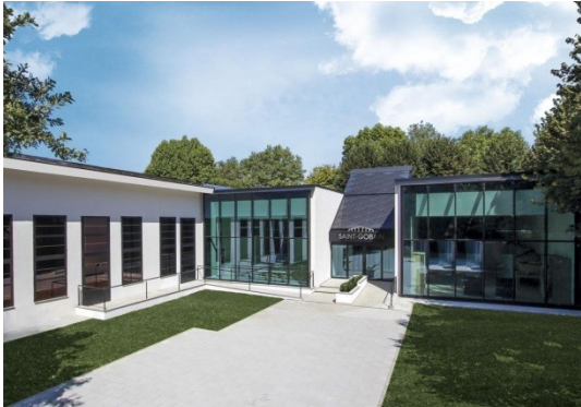
Innovation & training center in Italy, LEED Platinum, Primary energy need : 4,40 kWh/m 2 /anno
