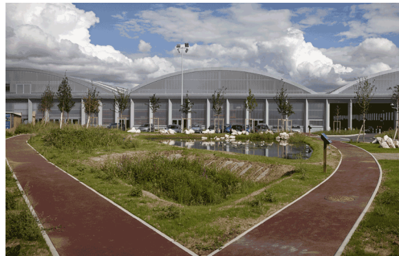
Halle de Pantin, undercover market, five times better than the requirements of the French RT 2012
